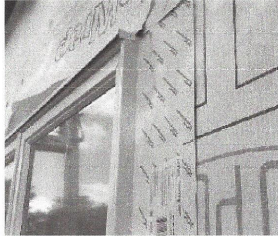
Proper Installation of Windows with Flange
